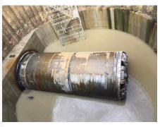
'Mary' our Tunnel Boring Machine (TBM), completes her 5km journey from Goxhill on the south side of the River Humber to the specially constructed shaft at Paull on the north bank.
