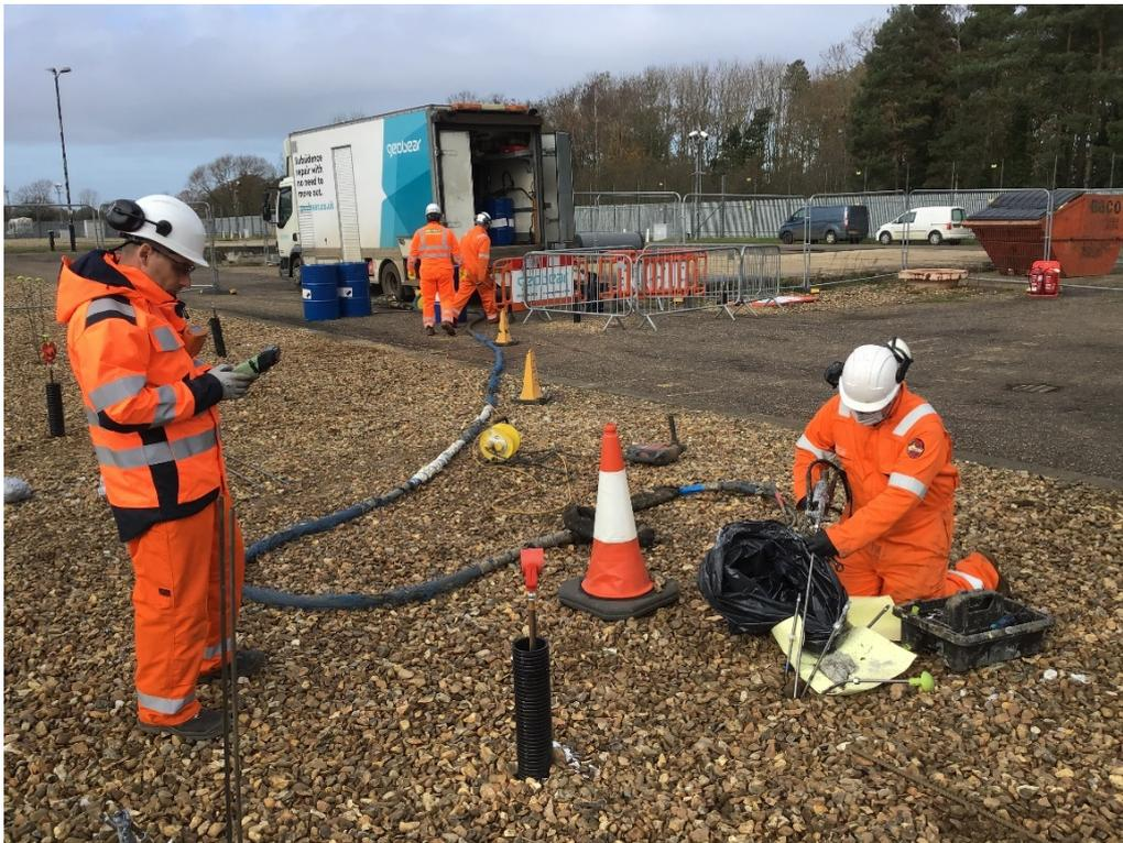
Figure 29 – Trial Geopolymer Injection
