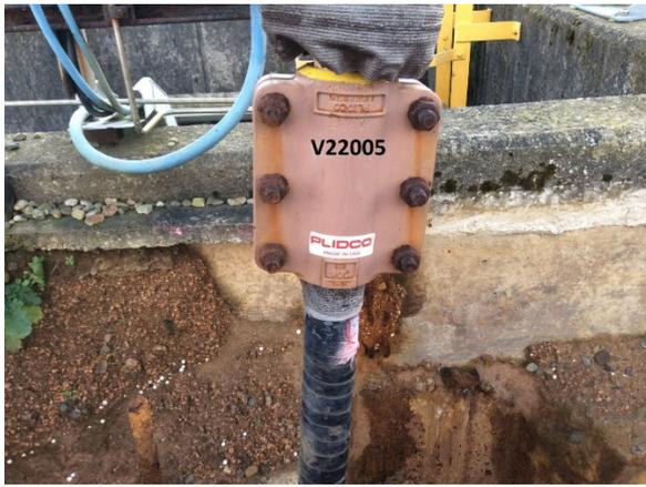
Figure 11: Temporary Plidco Clamp on Actuating pipework riser
