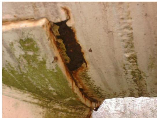
Figure 7: Corrosion under pipe support - a difficult failure to identify
