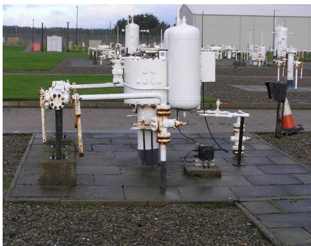
Figure 3: Typical gas-powered Actuator at St Fergus terminal
