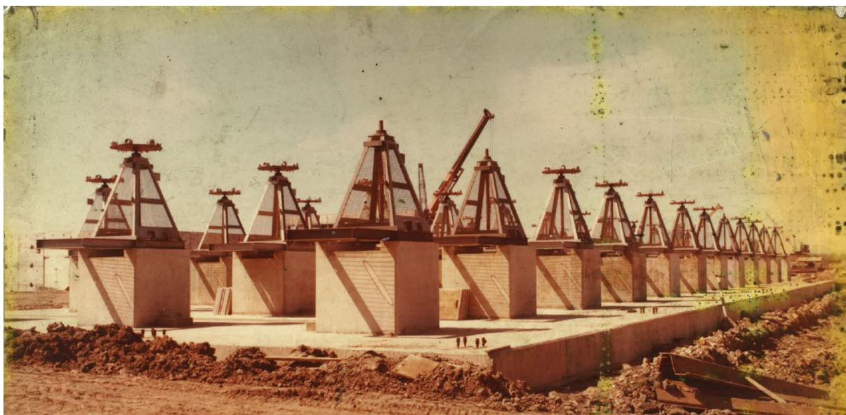
**Figure 10: Construction of Plant 1 Aftercooler (1974)**
