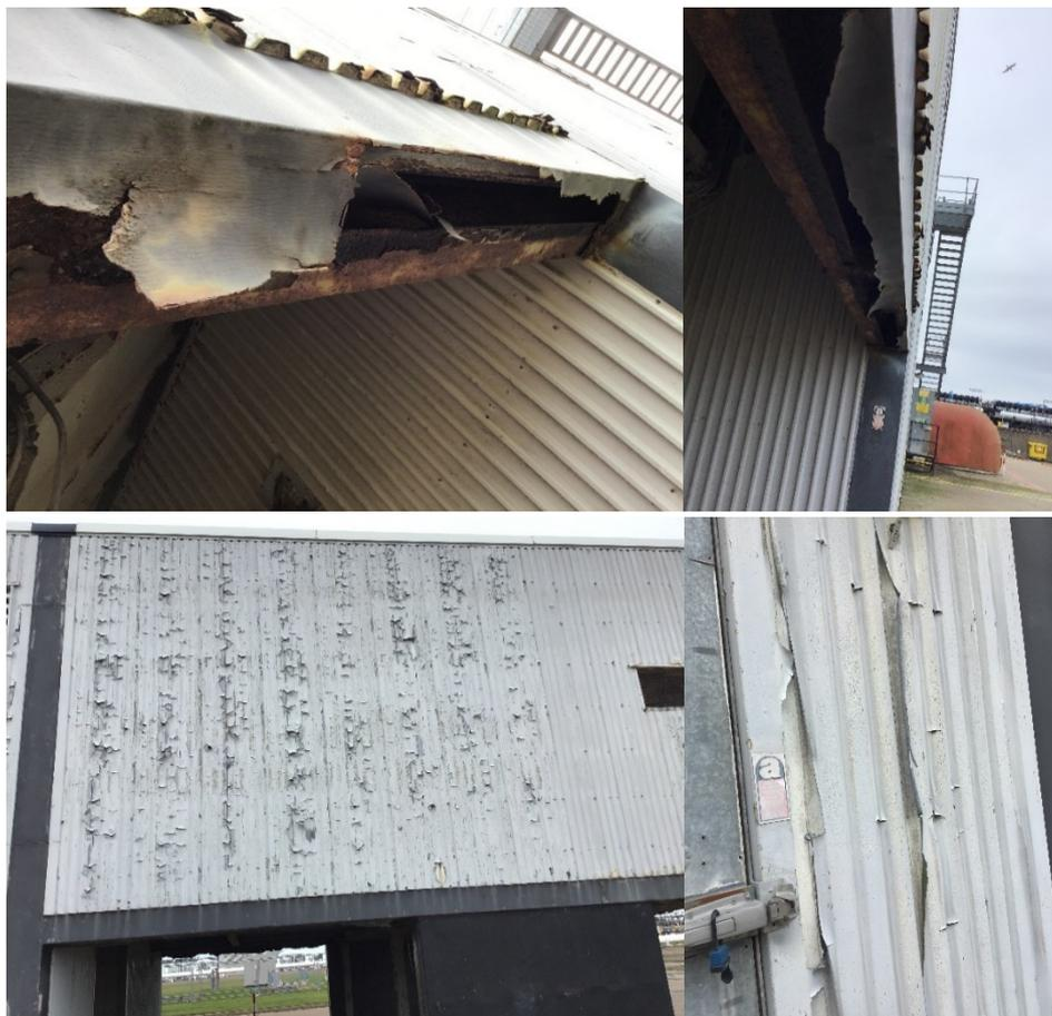
Figure 4: Coating breakdown of Galbestos cladding
