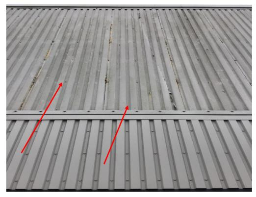
Figure 7: Flaking Cladding on 1B
