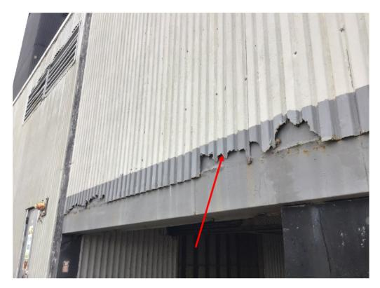
Figure 5: Flaking Cladding on 1C
