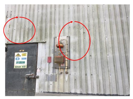
Figure 8: Flaking Cladding on 1D
