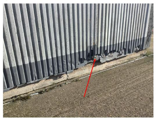
Figure 4: Damage on 1C Bottom Cladding
