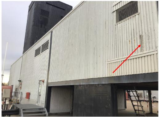
Figure 6: Flaking Cladding on 1A
