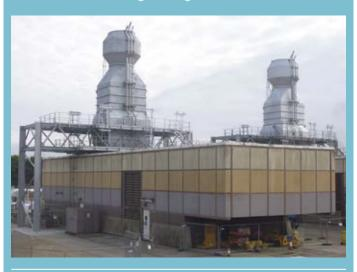
New exhaust stack and catalyst abatement system at Avlesburv comoressor station.
